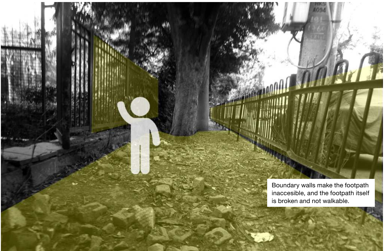
Figure 1.17: Inaccessible walking zone (Panchsheel Park South, New Delhi)
