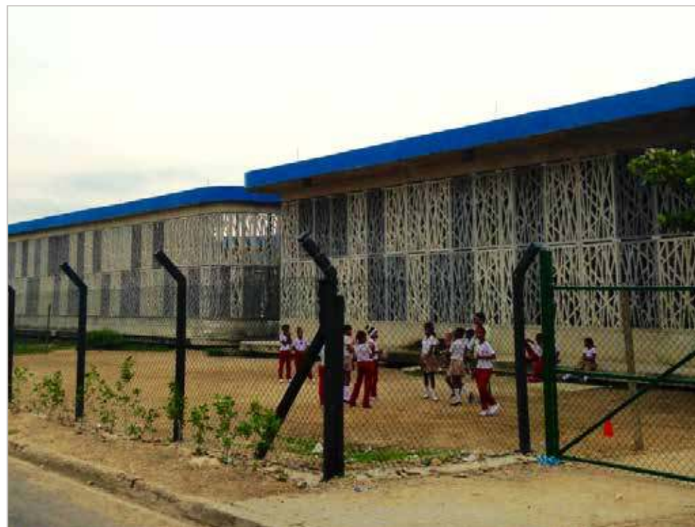
The makeshift football field next to the recently constructed school with subsequent fence
