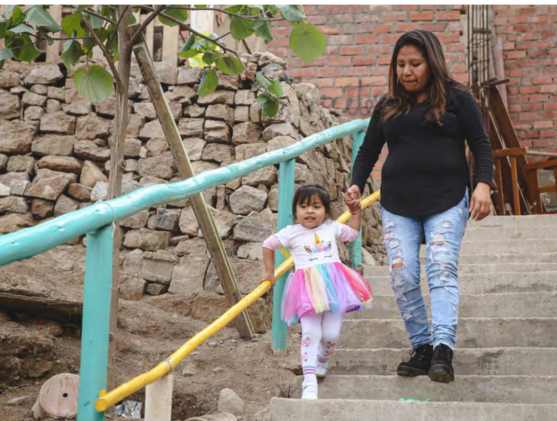
Adding a handrail at the height of a small child helps both the child and the caregiver navigate steps and feel safer walking. Lima, Perú. Source: Asociación Proyecto Alto Perú.
