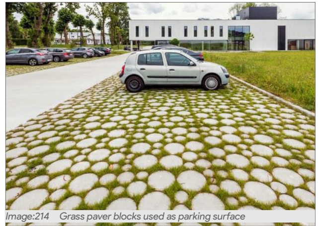
Image:213 Grass paver blocks used as parking surface
