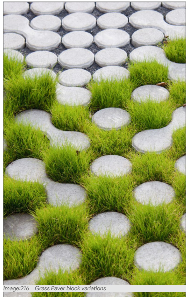
Image:214 Grass paver blocks used as parking surface
