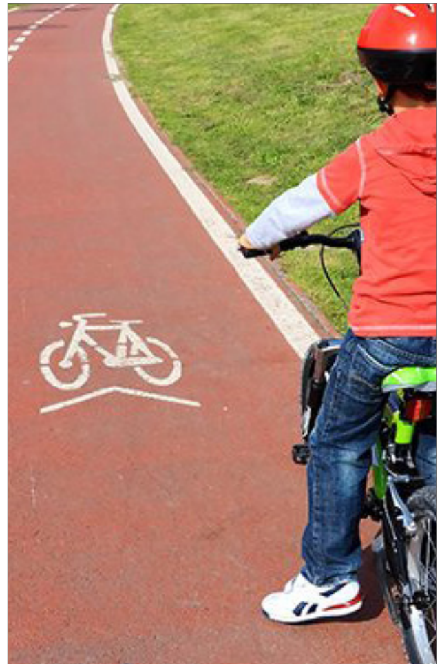
Image:268 Colored asphalt cycle track
