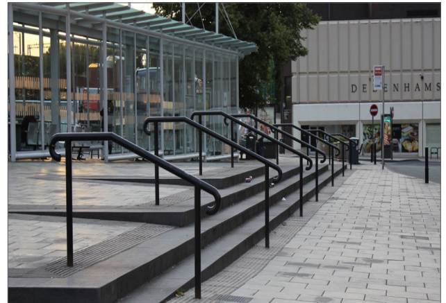
Image:160 Support at wide stairway
